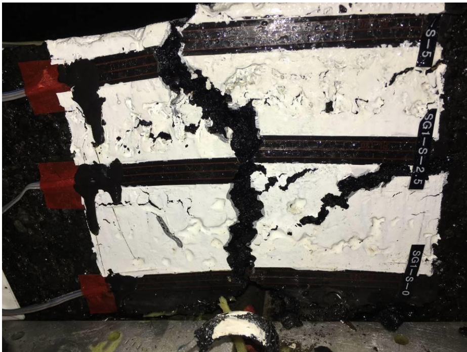
Fig 5 Bottom-up crack at inner vertical edge of south section reached top surface
