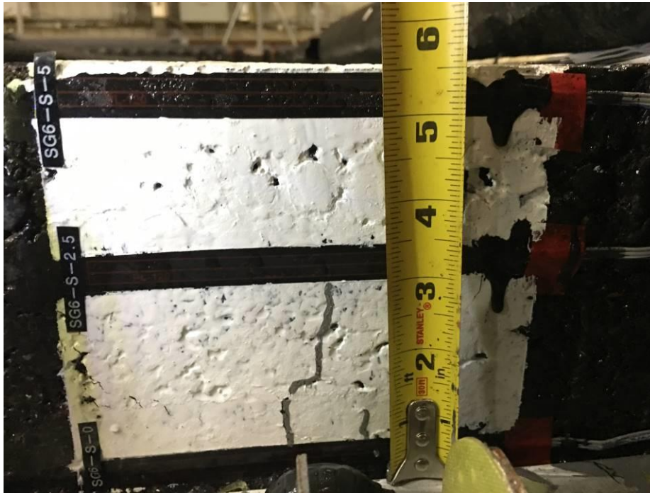
Fig 6 Bottom-up crack at SG6-S-0 3 inch long
