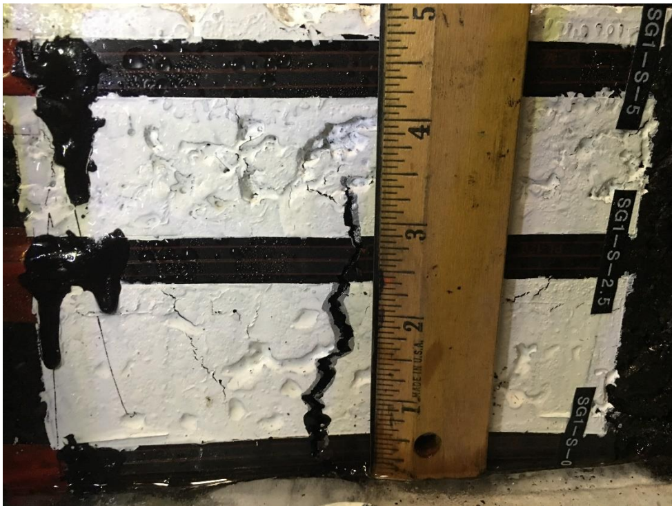
Fig 4 Bottom-up crack at SG1-S-0 3.5 inch long
